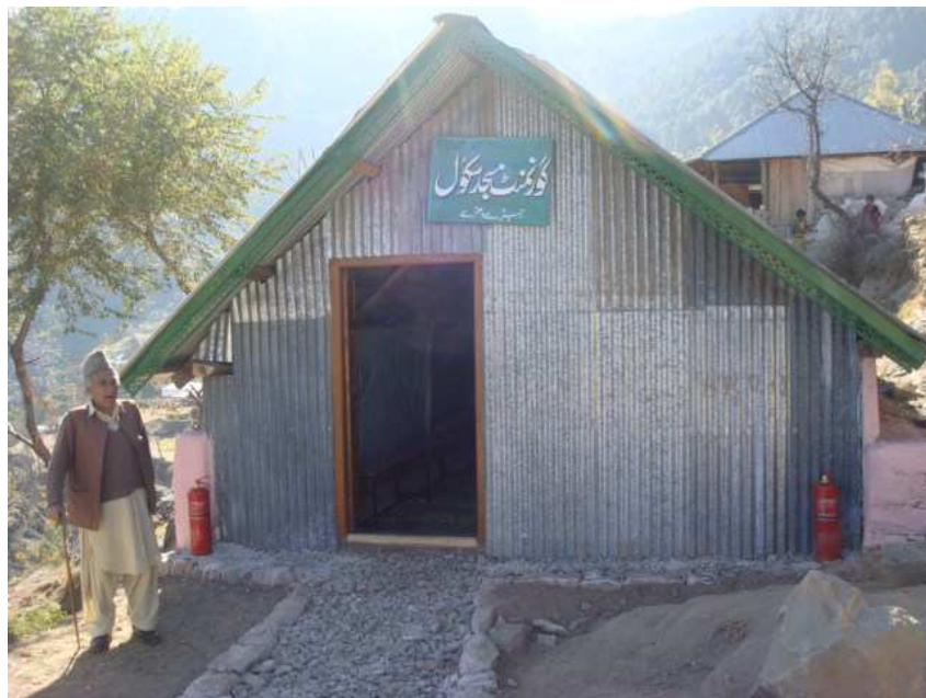
Government Masjid Maktab School Jabray Dharray in Bagh used a RISE grant to construct a temporary shelter for the school
